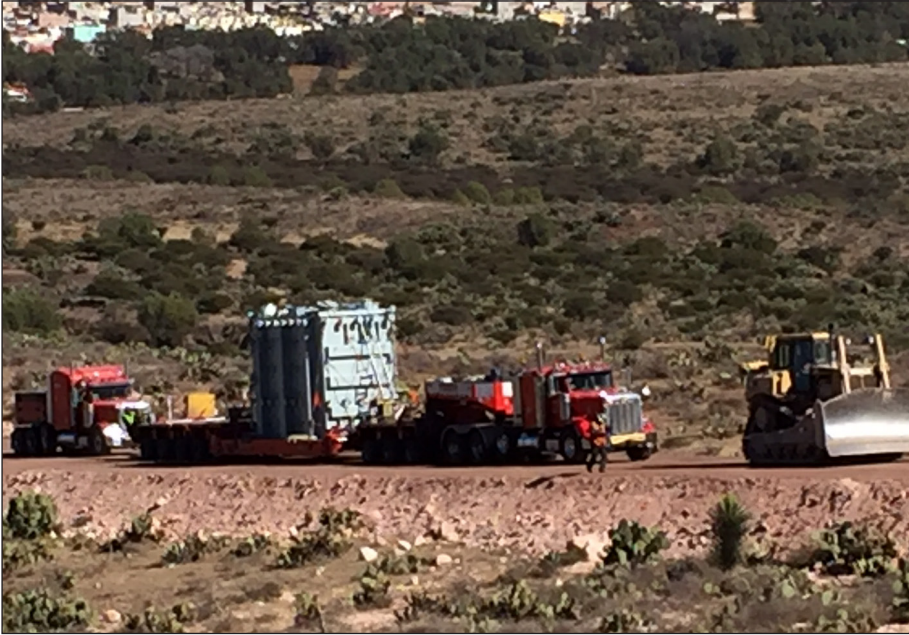
Engineers slowly guide a substation for the 130 MW La Bufa Wind Farm up a steep incline.
